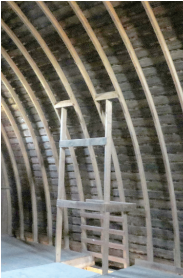
Courtesy of Dennis Kingery Laminated rafters
