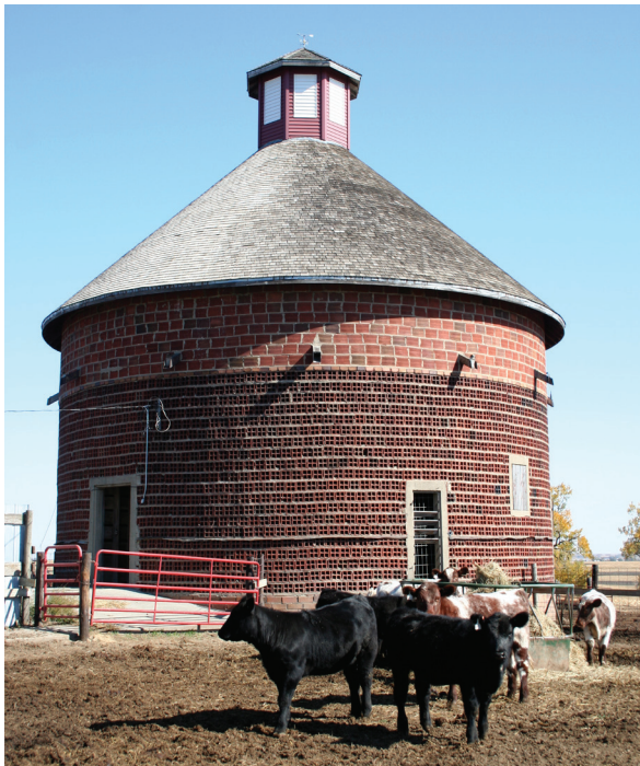
Harrison County 3322 Overton Avenue, Logan
