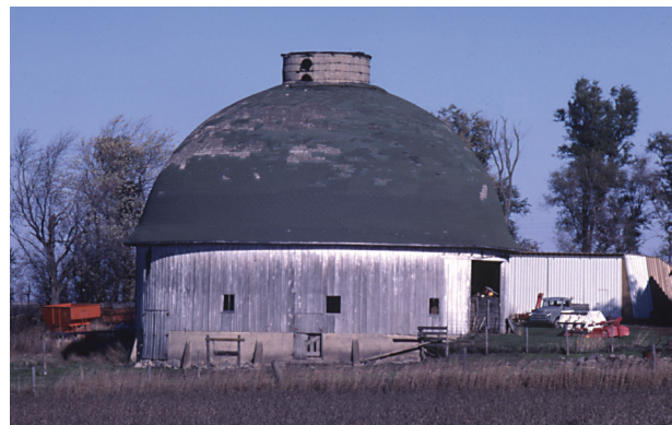
Barn before moving and restoration
